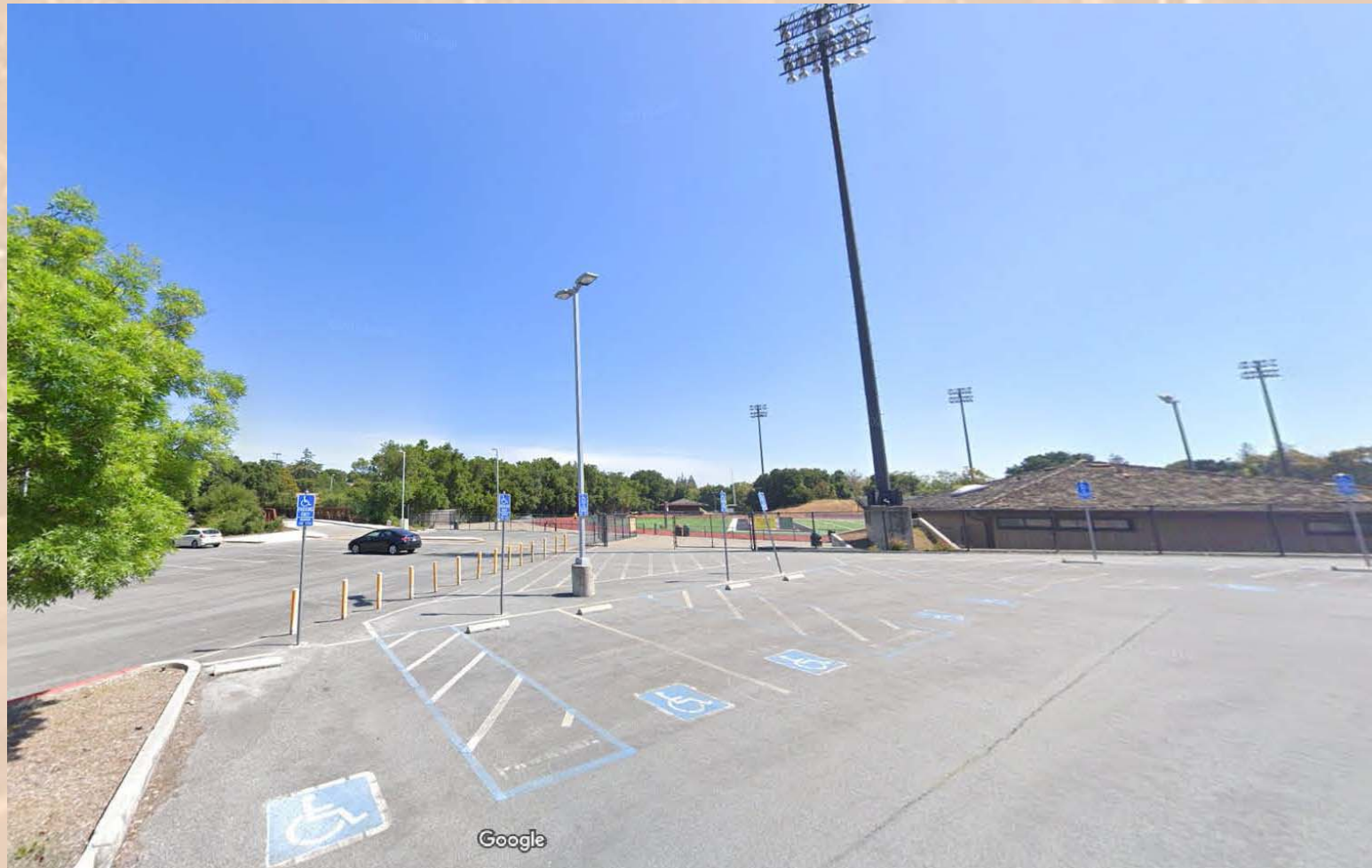
Accessible Parking Stalls in Lot 1
